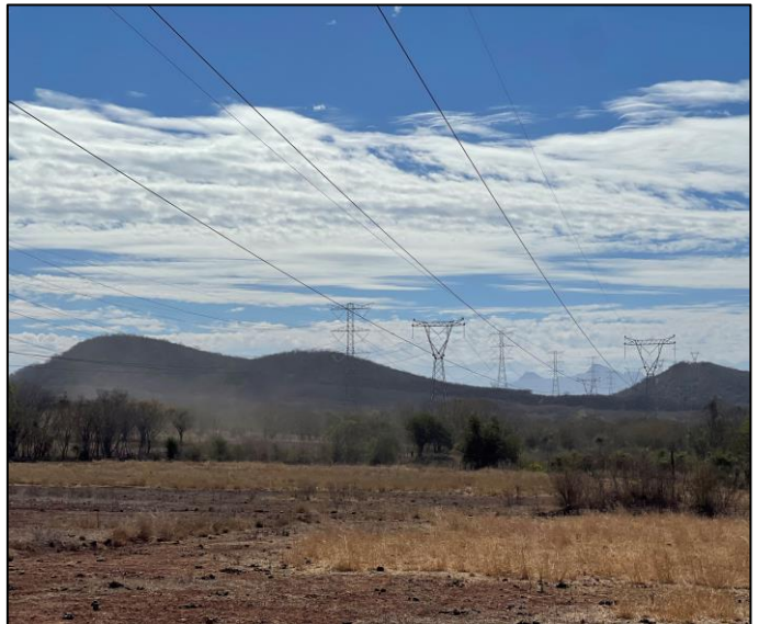
High voltage national grid near site
